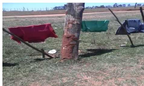
Fig. 5b: Termites on a fencing pole
