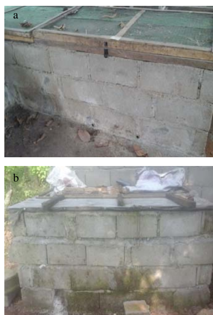
Fig. 3(a-b): Trench pens
